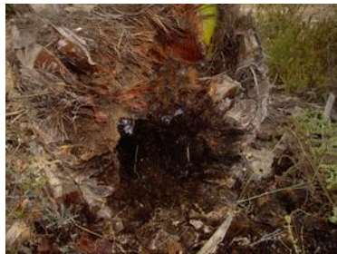
Palm 9468 daños base (31-08-1
